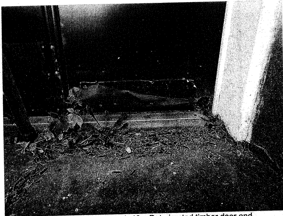
PHOTO NO. 1.43: Routine Repair 18 – Deteriorated timber door and frame – North Elevation, Grid 2-3: Ht. 0' +/-
