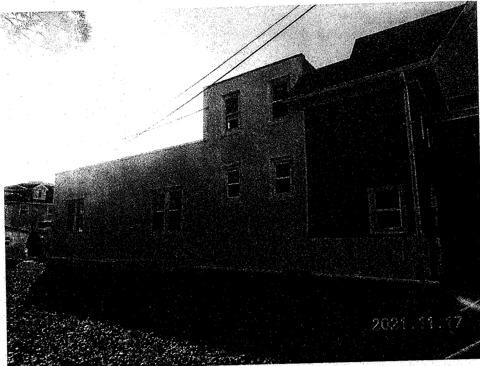
PHOTO NO. 1.3: General View – East Elevation
