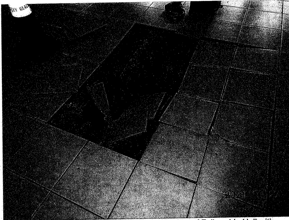
PHOTO NO. 1.23: Priority Repair 7 – Overall view of Fellowship Hall with failing floor system due to severely deteriorated timber stringers and subfloor – Lower Level, Grid A-E/2-4
