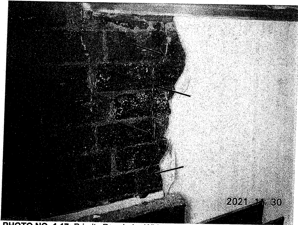
PHOTO NO. 1.17: Priority Repair 4 – Wide vertical crack in unreinforced cinder block wall of the Gymnasium – South Elevation, Grid 1-5: El. 0'-20'+/-
