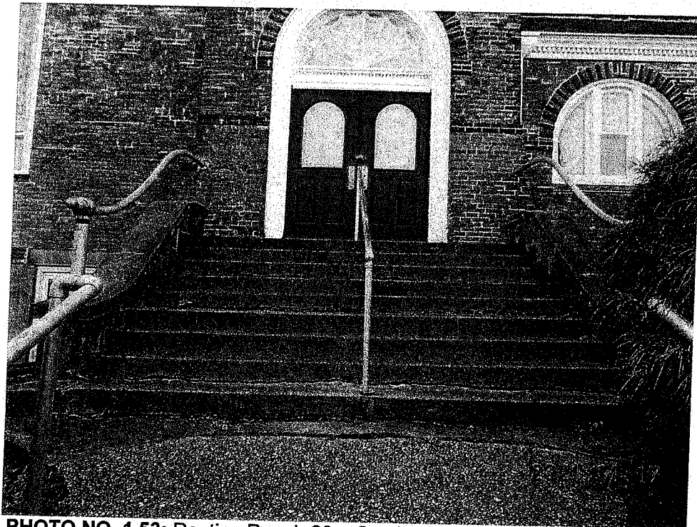
PHOTO NO. 1.53: Routine Repair 28 – Cracked and detached concrete stair treads – Site, Grid A.0-A/4-5
