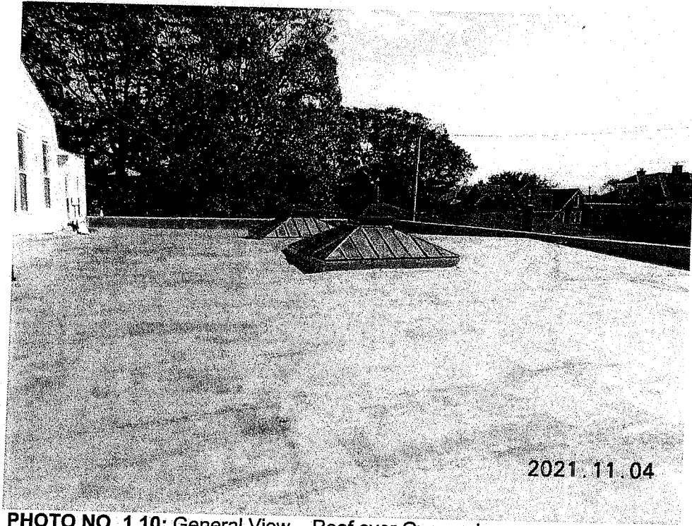
PHOTO NO. 1.10: General View – Roof over Gymnasium
